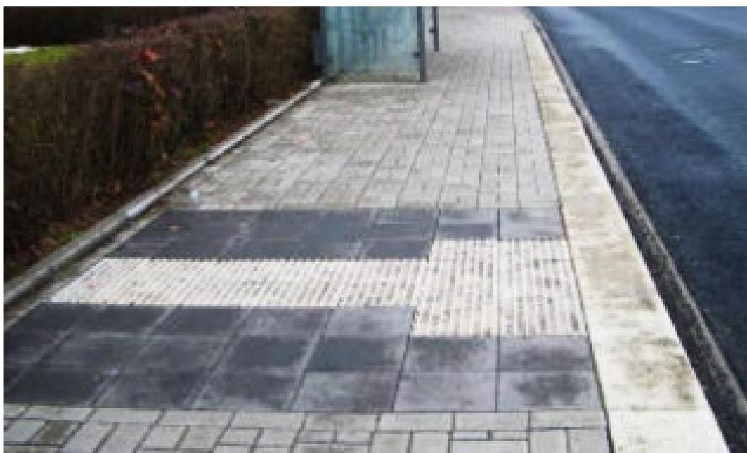
*Figure 6. The layout of tactile surfaces on a bus stop platform in Germany.*
