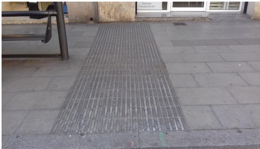
*Figure 8. The layout of tactile surfaces on a bus stop platform in Spain.
