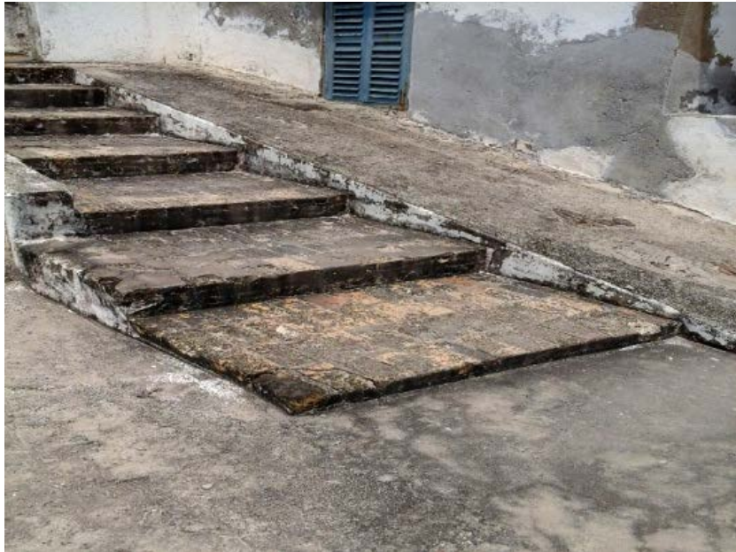
Figure 1. The entrance of Cape Coast. Source: Field Photovoice (2015).
