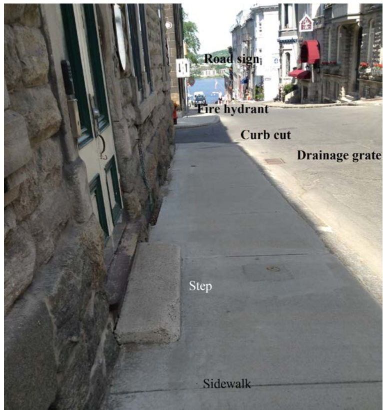
Figure 2. Example of a street section observed in Quebec City
