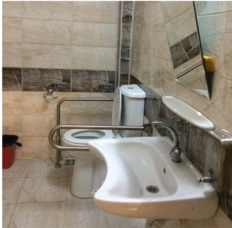
Figure 9. Building B toilet
