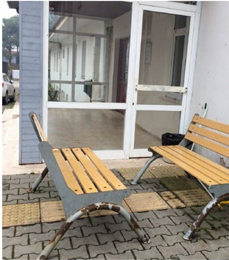
Figure 6. The main entrance of building A (music department block)
