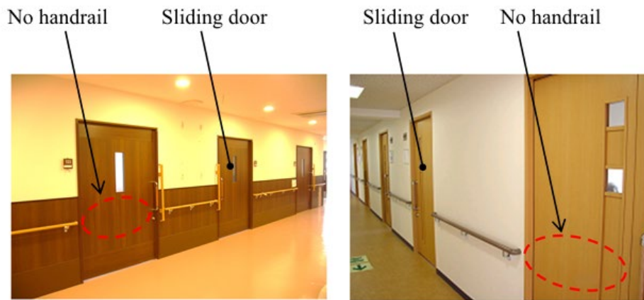
Figure 1. Examples of sliding doors used in Japanese welfare facilities.
