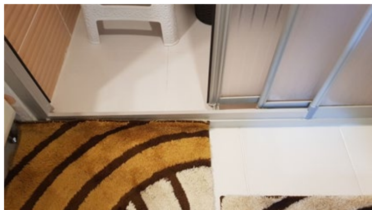
Figure 3. The shower threshold causing trouble for the user with MS
