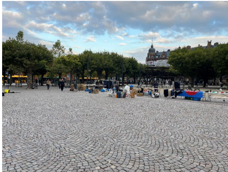
Figure 1: After the reconstruction of the square the area is covered by uneven street stones without contrasts.
