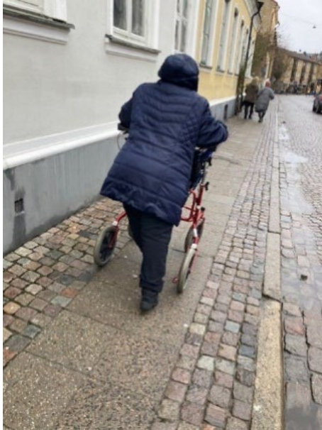
Figure 3: The walkway has a steep side slope, putting users in danger of falling, especially when using a walker or wheelchair.
