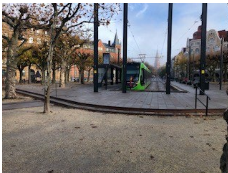
Figure 2: A new level difference with stairs was created in an earlier flat area, when constructing the new tram station.
