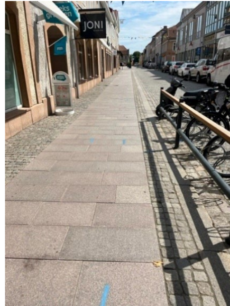
Fig 6. One example of how ground surfaces have been improved in connection to the city's maintenance work. The uneven street stones are now only decoration on the sides of the walkway.
